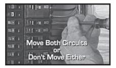
When three-conductor wiring is used, two 120 volt circuits will often share the same neutral wire. To avoid overloading the neutral, you should either move BOTH of the circuits that share the neutral or don't move either of them.
